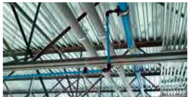
Alternative energy Transair Ø 76 and Ø 63
