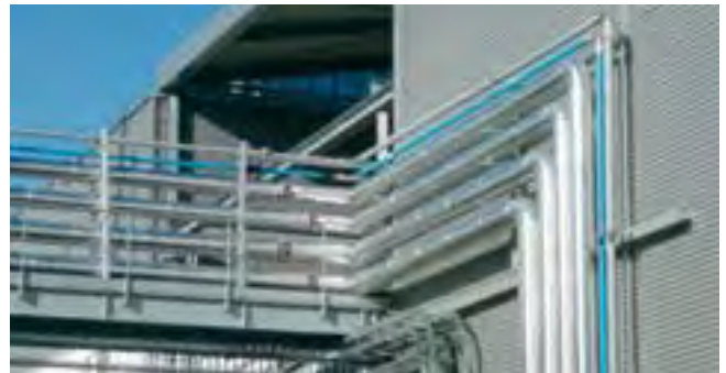
Outdoor installation Transair Ø 168
