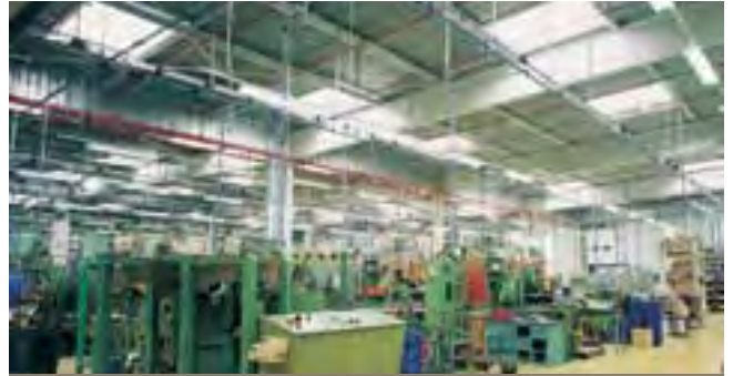
Assembly workshop Transair Ø 63 and Ø 25
